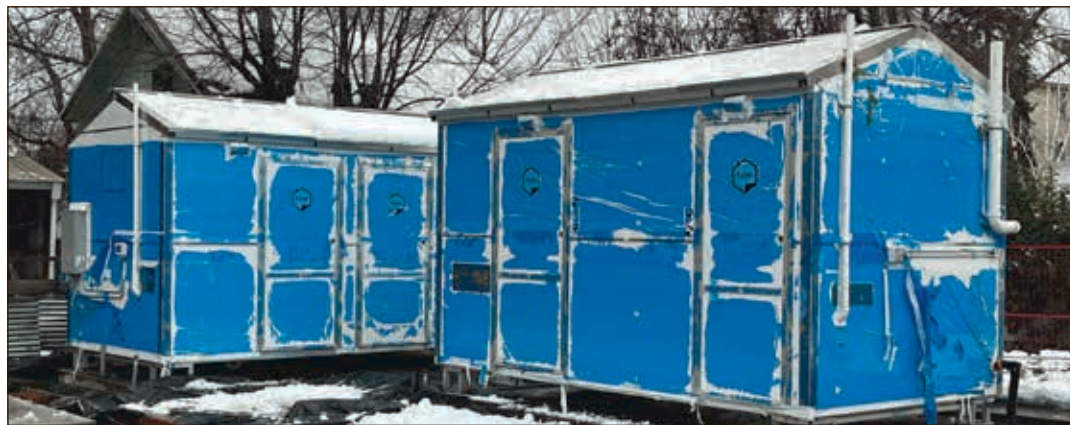
A transitional emergency shelter downtown Klamath Falls is being built and includes tiny houses. It is the first shelter the Klamath Tribes has operated, and the first of its kind in Klamath County. (Ken Smith/Klamath Tribes News)
