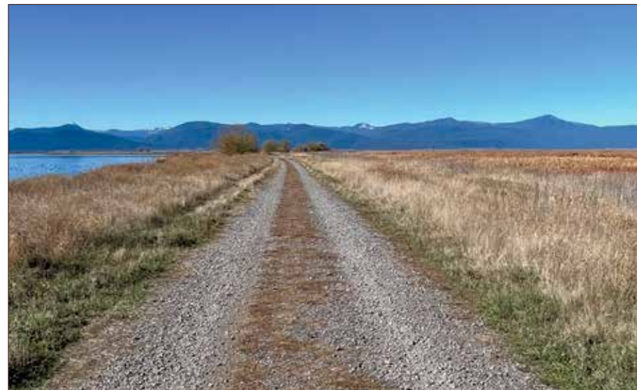
An approximately 7-mile man-made levee passes through wetlands adjacent to Agency Lake, with more soon to be added as part of the Agency-Barnes Units wetlands project overseen by the U.S. Fish and Wildlife Service. (Ken Smith/Klamath Tribes News)
