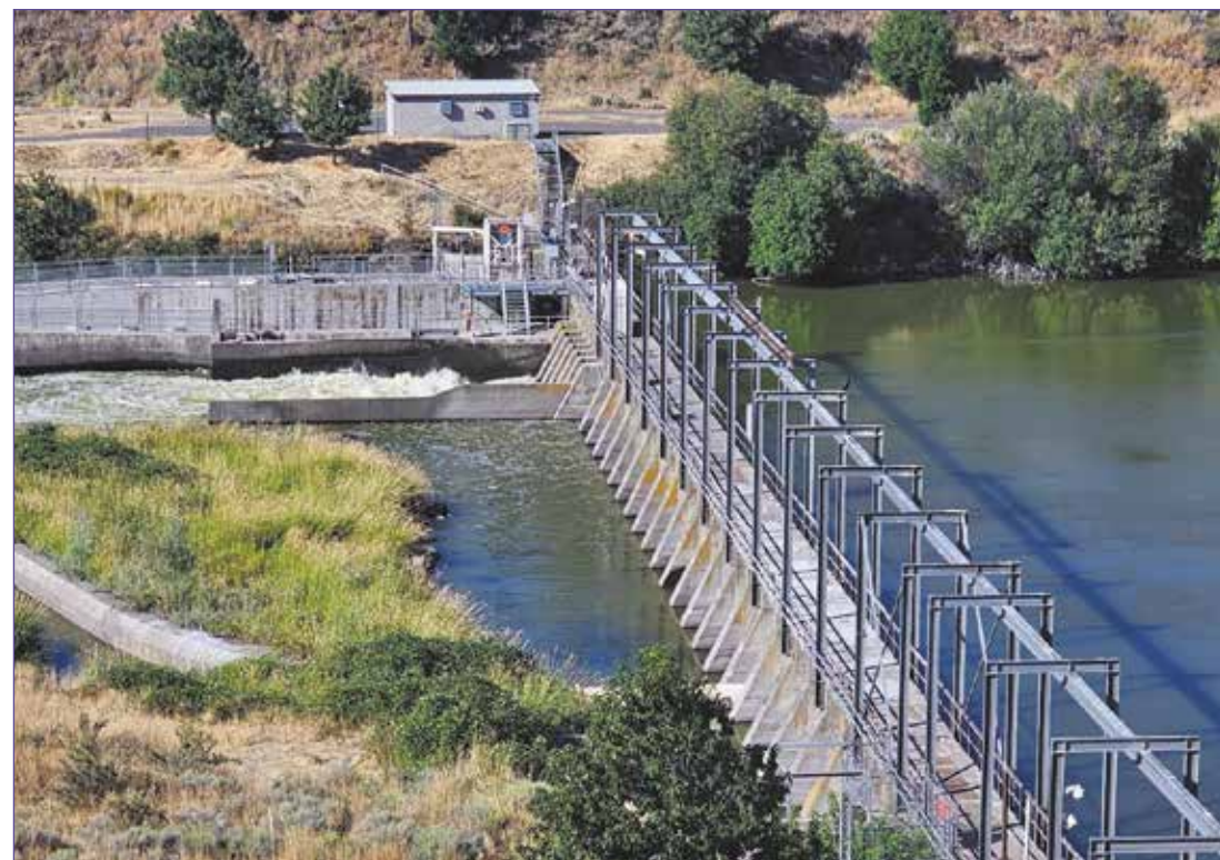
The Link River Dam is viewed from Conger Heights Park. On the far bank, the fish ladder and control house above it can be seen. (Christopher German/Klamath Tribes News)
