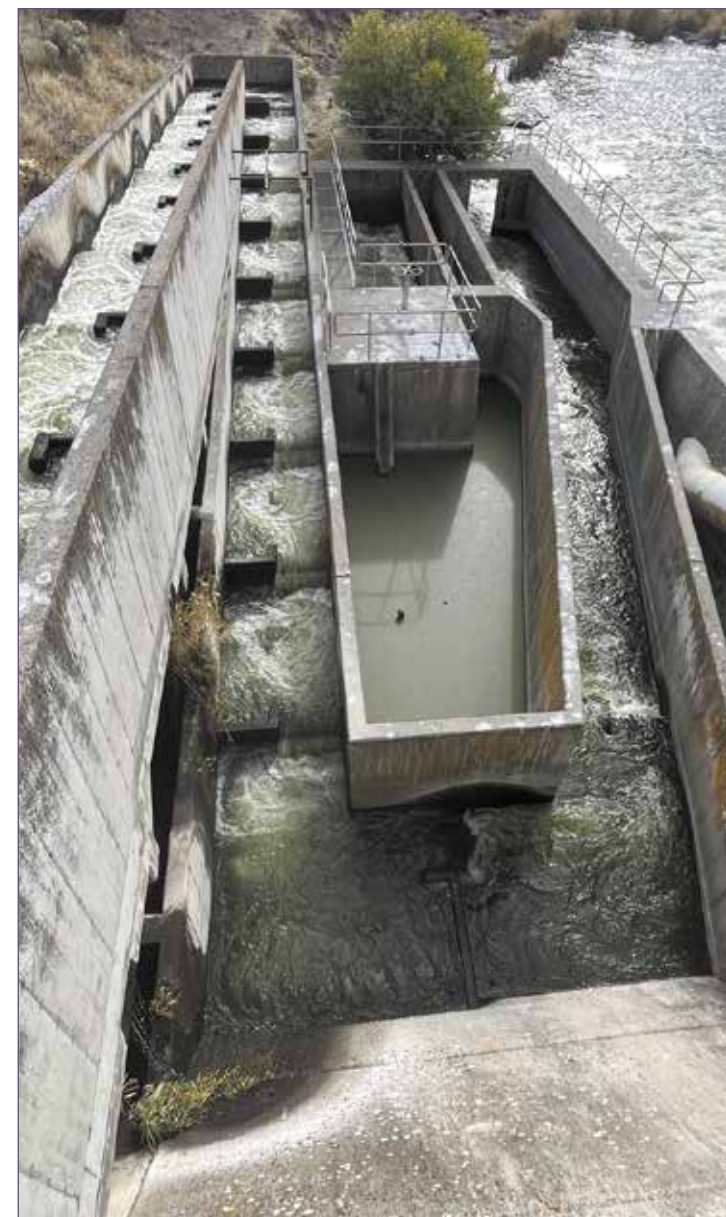
The Keno Dam fish ladder is in question regarding its ability to accommodate migrating salmon. (Ken Smith/Klamath Tribes News)
