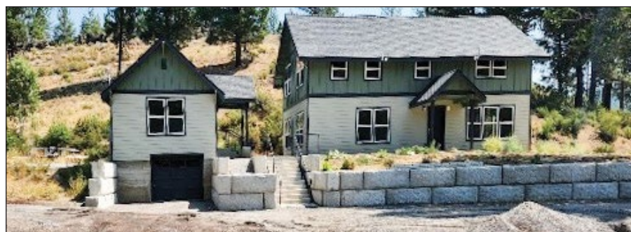
New facilities built at Ambodat to house the growing workforce and expanded capacity.
